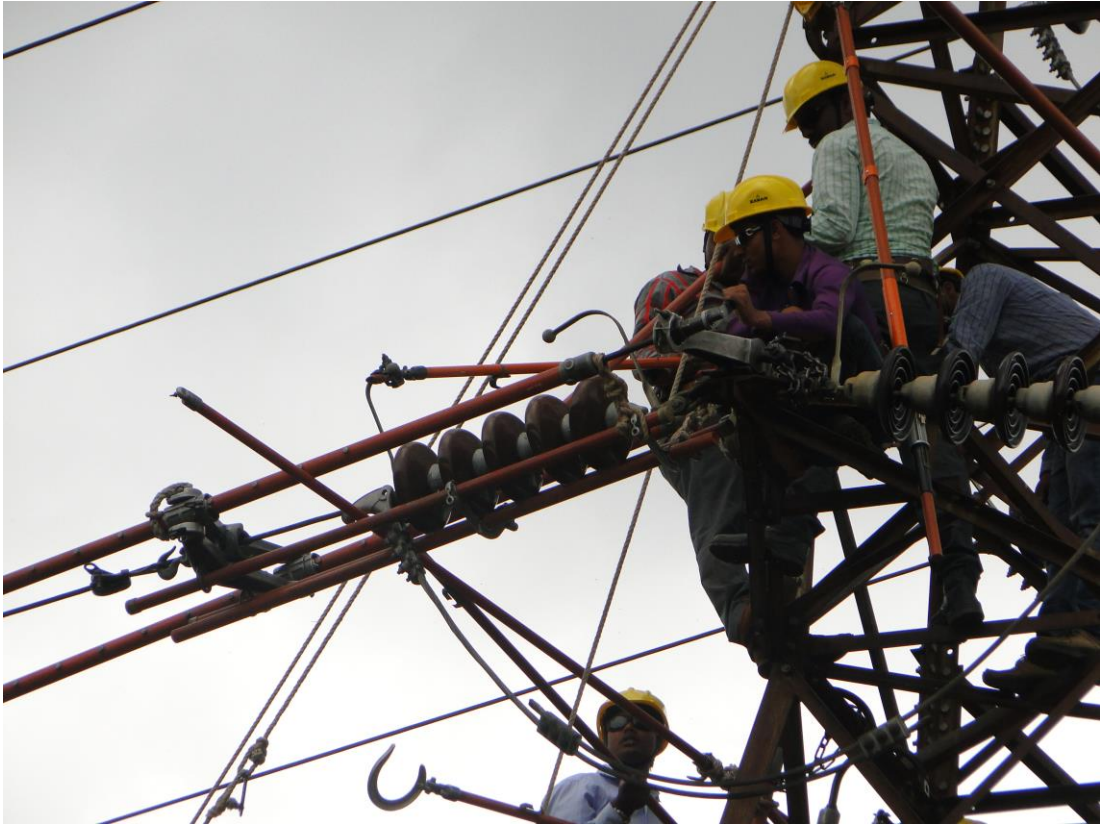
66KV Tension Operation
