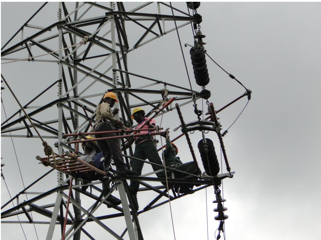
110 KV Tension Operation
