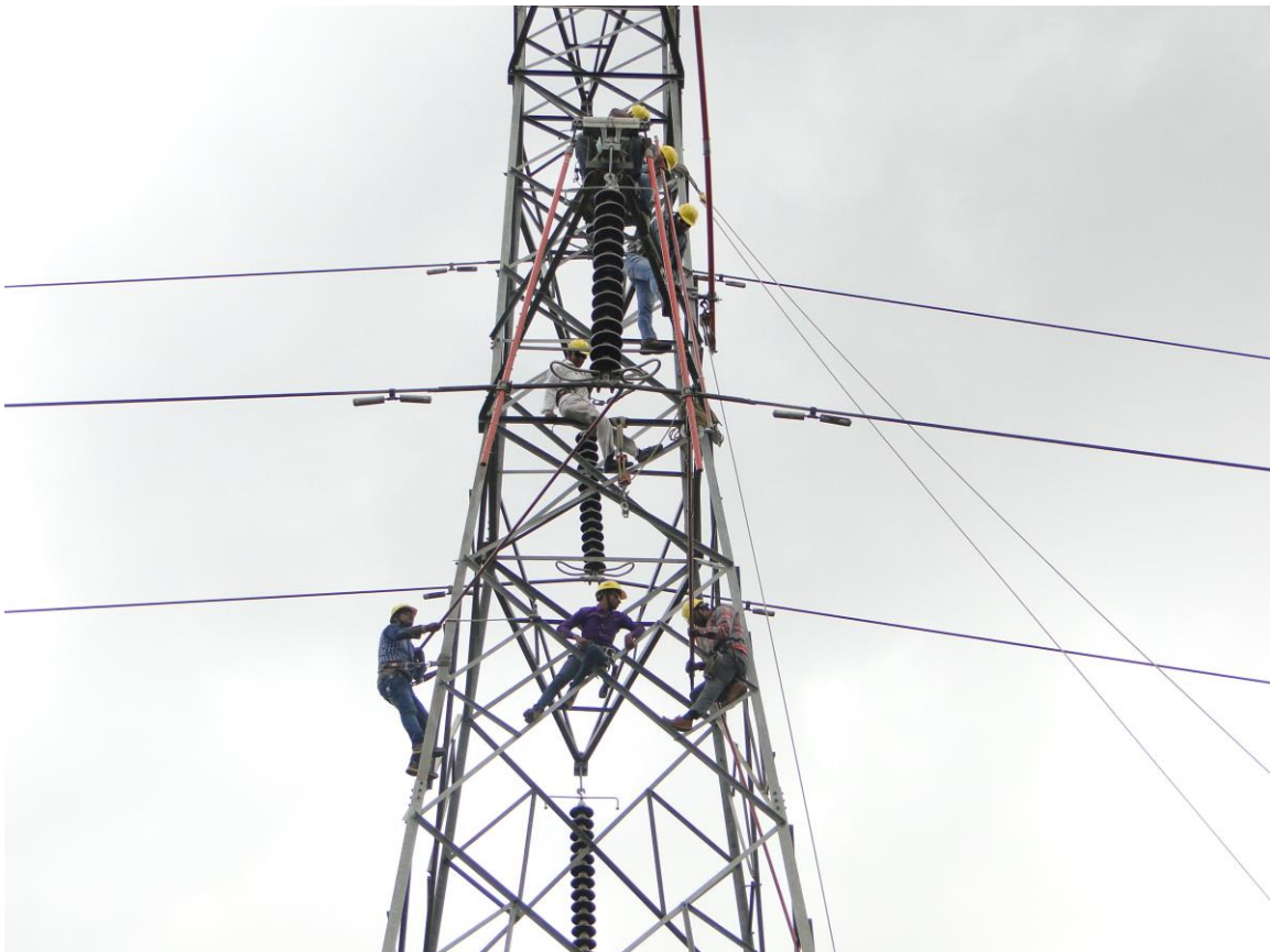
220 KV Suspension Operation
